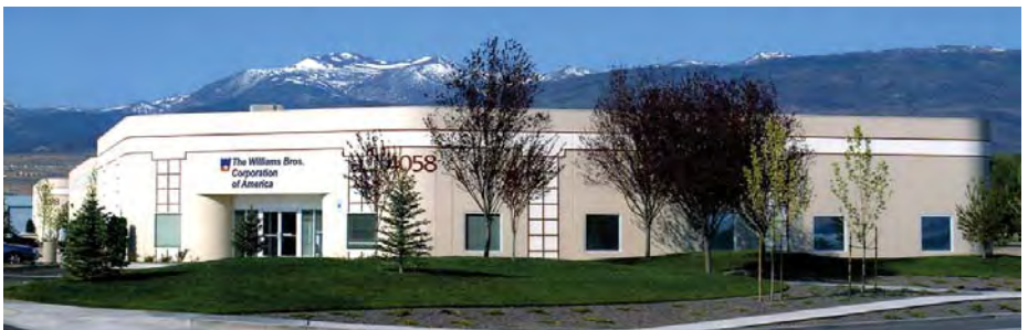
Western Distribution Center, 4058 S. McCarran Blvd., Bldg. A, Reno, NV 89502
